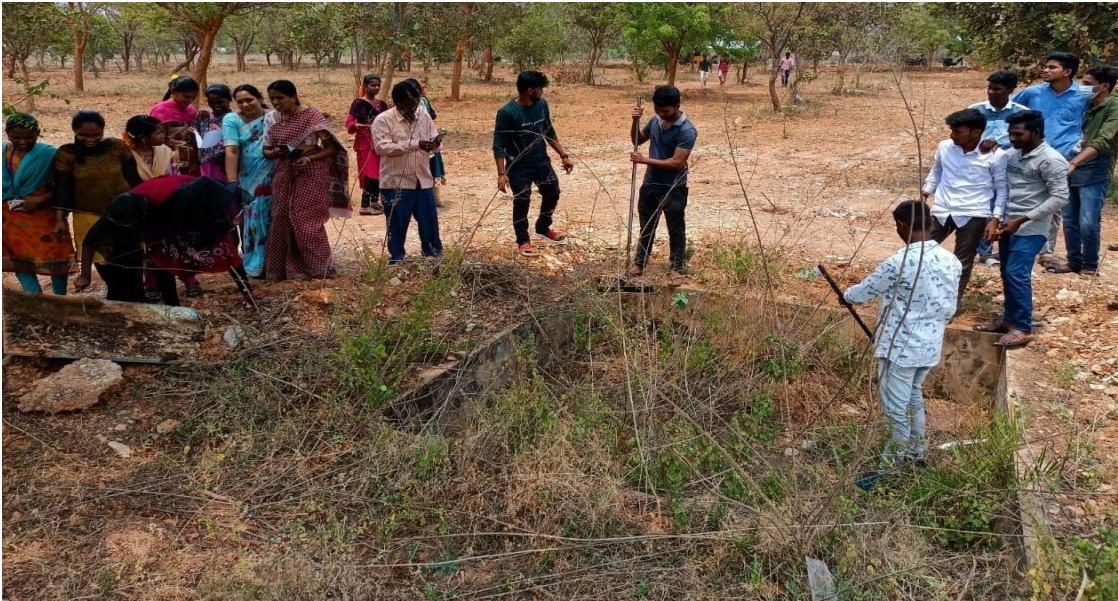
RainWaterHarvestingpit before cleaningbyNSSVolunteers.
