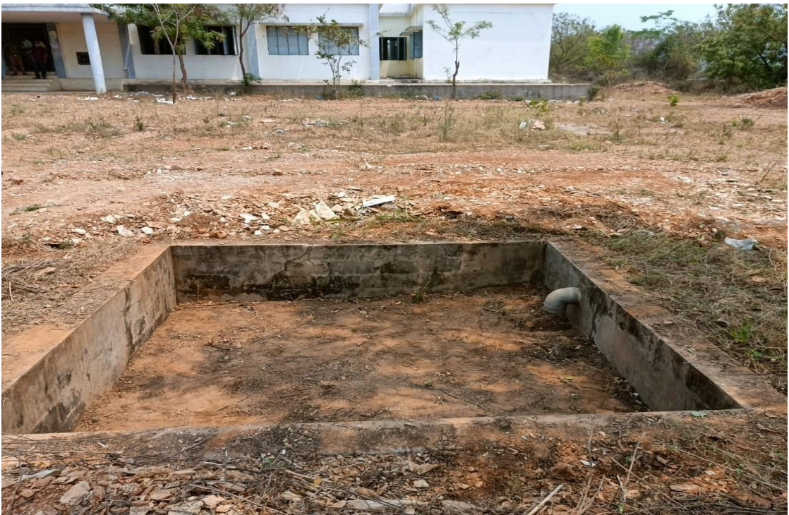
Rain Water Harvesting pitaftercleaningbyNSS Volunteers.
